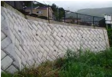
Fig.5 Example of Kenchi blocks retaining wall
