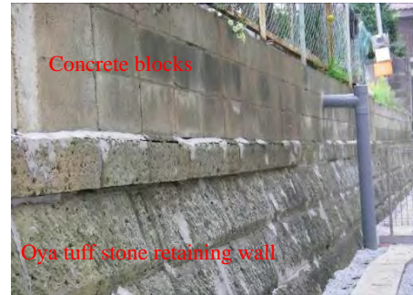
Fig.10 Example of Oya tuff stone retaining wall
