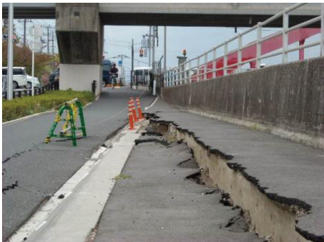
Photo.3 Difference of sidewalk height (right side: old levee) (Imagawa area)
