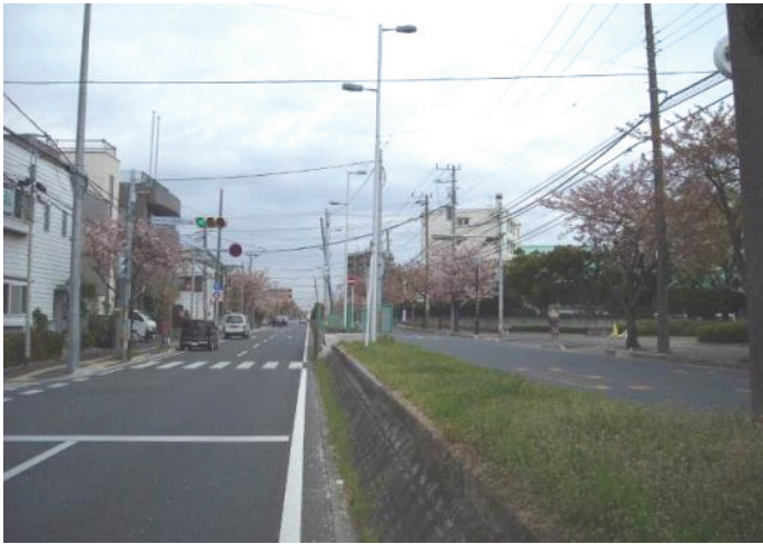
Photo.6 Boundary of newly reclaimed land and old residential areas in the Route 357 (small retaining wall just located in the center)
