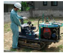
Photo 1 Overall view of measuring the underground water level
