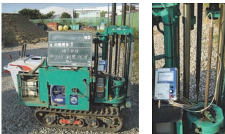
Fig. 1 Measurement of groundwater level using the SWS test hole in progress
